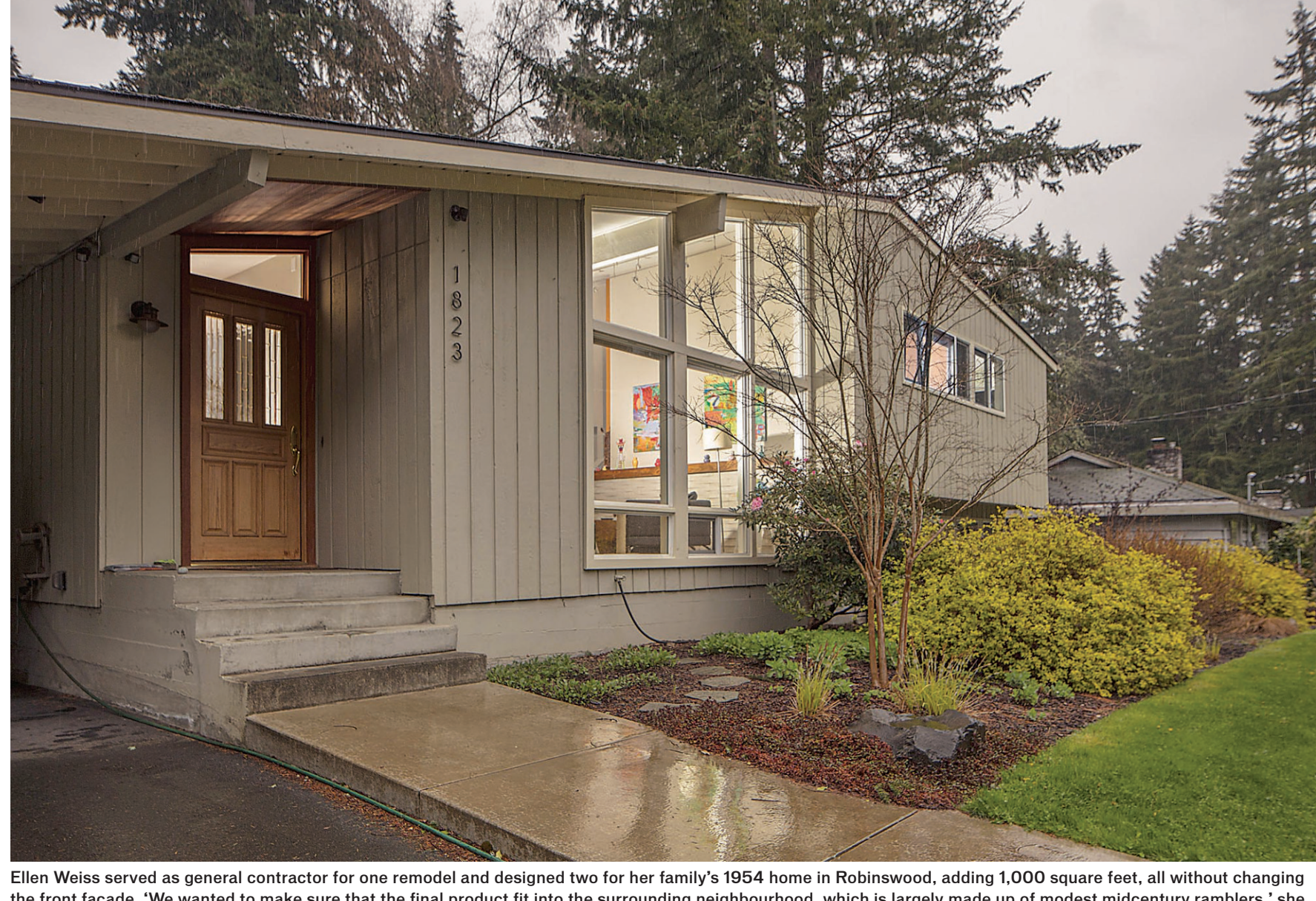
Ellen Weiss served as general contractor for one remodel and designed two for her family's 1954 home in Robinswood, adding 1,000 square feet, all without changing the front facade. "We wanted to make sure that the final product fit into the surrounding neighbourhood, which is largely made up of modest midcentury ramblers," she says. PHOTO: STEVE RINGMAN/TRIBUNE NEWS SERVICE
